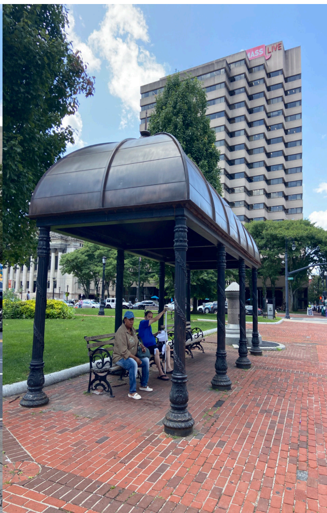
Figure 16: Bus shelter and sidewalk in good condition in Springfield.
