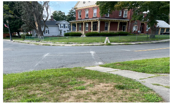
Figure 10: Poorly visible crosswalk in South Hadley study area.
